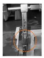
1) Frame Stanchion bracket, with stanchion secured by peg and cotter pin.
